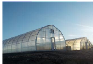
Polycarbonate (PC) greenhouse, active ventilation, storage system and unheated. Kuujuaq, Nunavik
